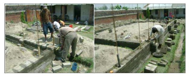
Figure 22 Block work at second layer and laying of U-block for plinth ring beam
