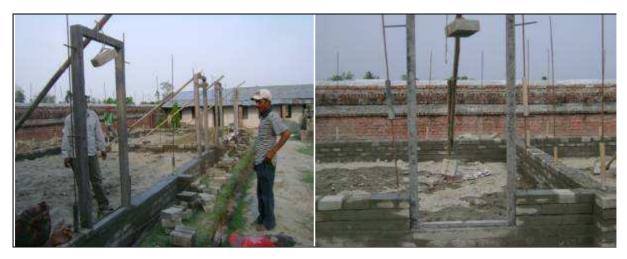
Figure 24 installation of door at plinth level
