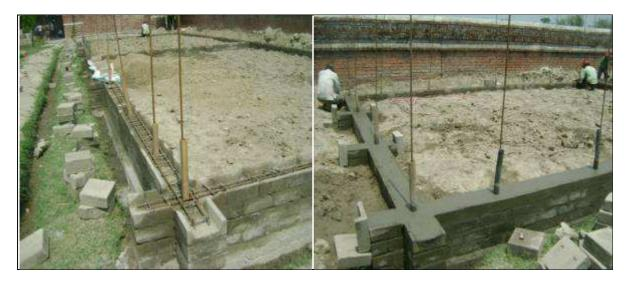
Figure 23 arrangement of reinforcement and concreting of plinth ring beam
