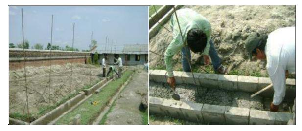
Figure 19 arrangement of vertical reinforcement and concreting of foundation ring beam
