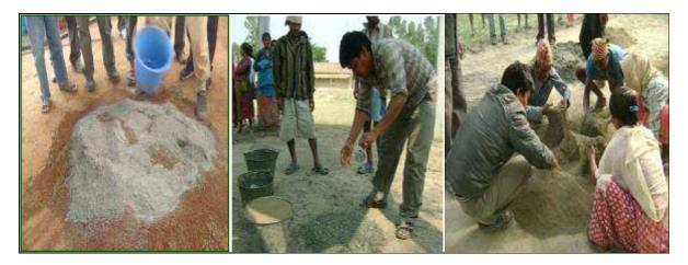
Figure 12 soil and cement mixing, sand and water mixing, and together mixing at Morang district
