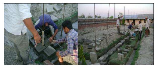
Figure 21 Starting of block work at first layer
