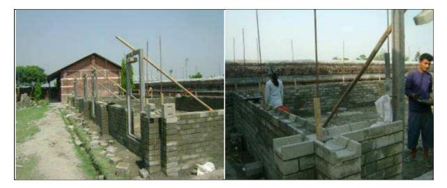
Figure 25 sixth layer from plinth level and arrangement of U-Block for sill ring beam
