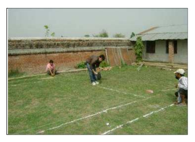
Figure 15 layout for excavation of foundation at Morang district
