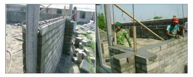
Figure 26 arrangement of reinforcement and concreting of sill ring beam
