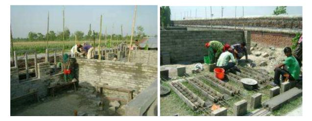
Figure 28 block work at corner tie and preparation of lintel
