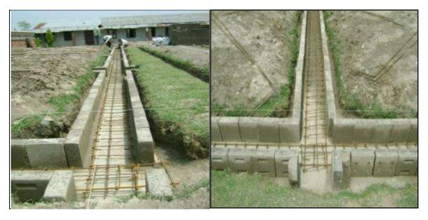
Figure 18 Framing and arranging reinforcement for concreting of foundation ring beam
