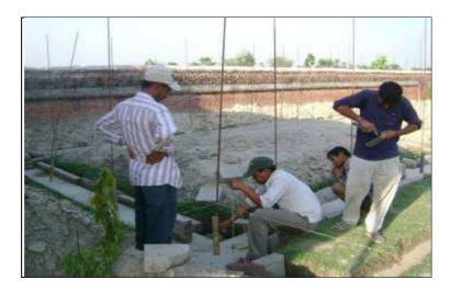
Figure 20 Completion of foundation ring beam
