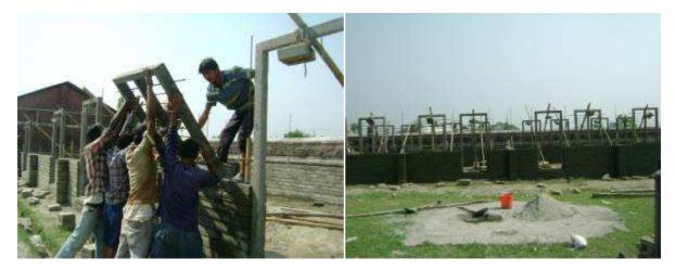
Figure 27 installation of windows above the sill ring beam
