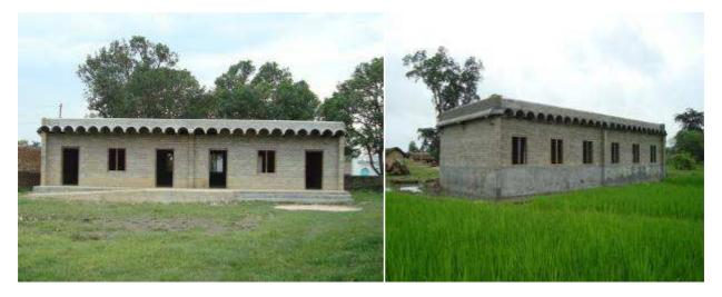
Figure 30 Ferro Cement Channel roofing system at bake district
