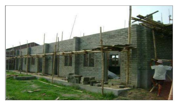
Figure 29 completion of lintel ring beam
